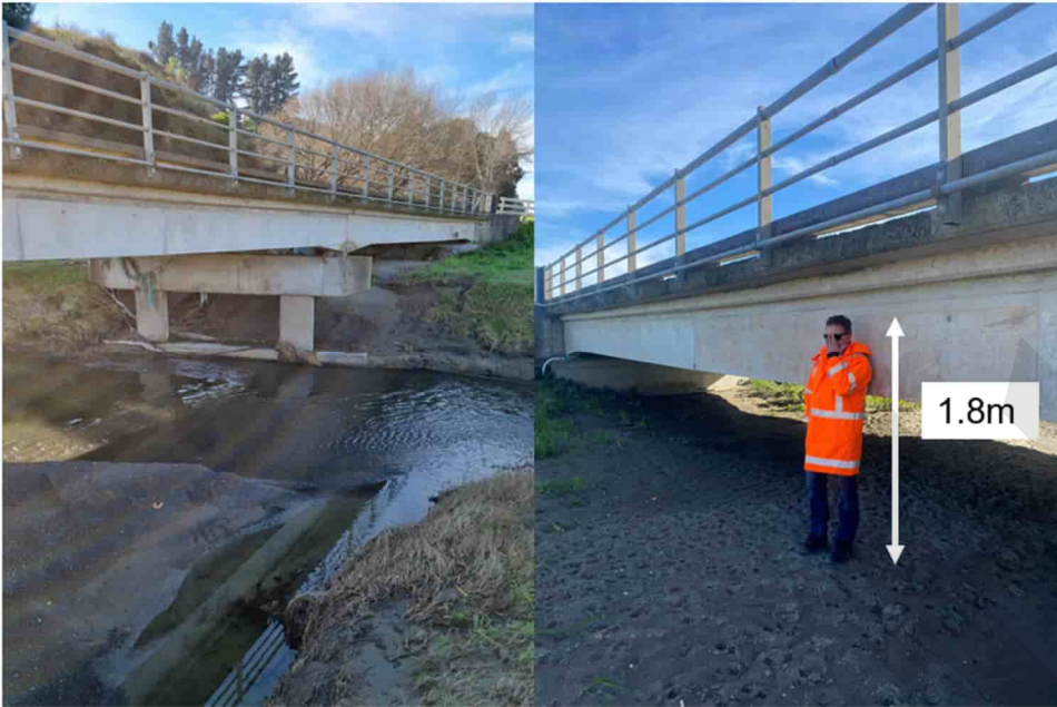
Figure 4.4 Taihape Road bridge
