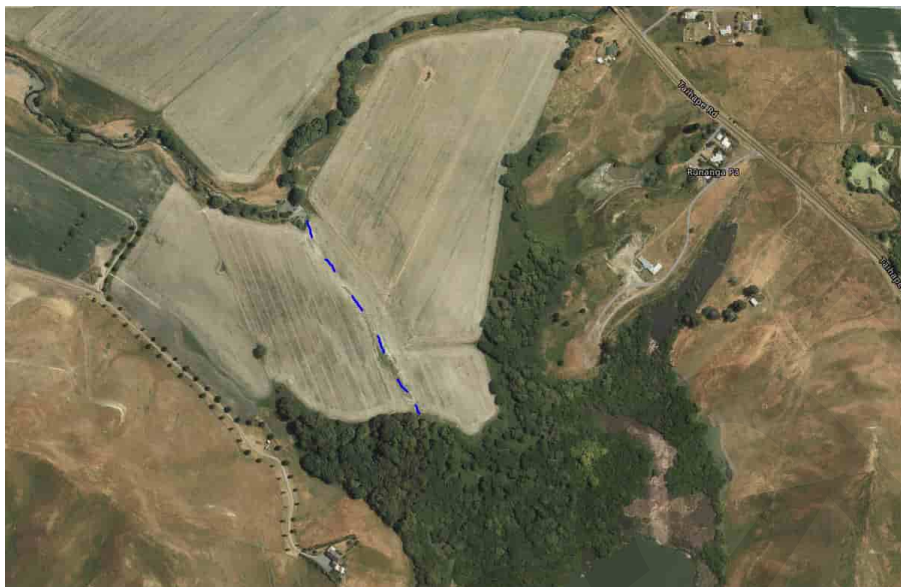
Figure 2.2-High flow spillway into Lake Runanga
